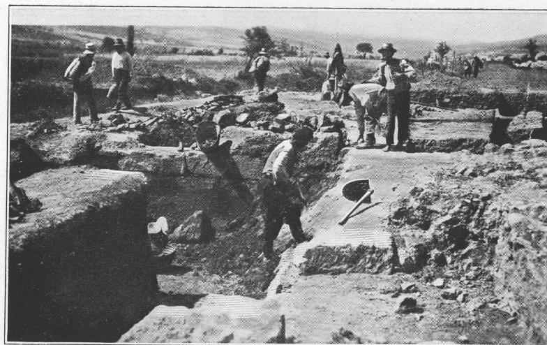
Cross wall in west section of the Gymnasium—from the south.
